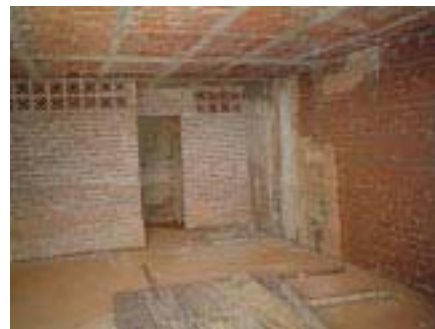
The facilities Before
